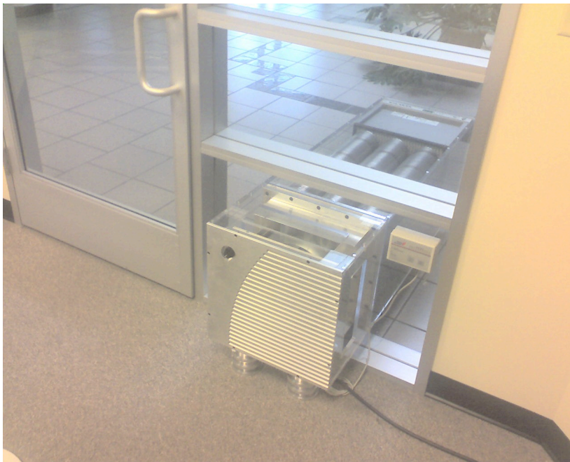
Caption: The Aero Guardian fan is inside the protected area and the filtration system remains outside.
